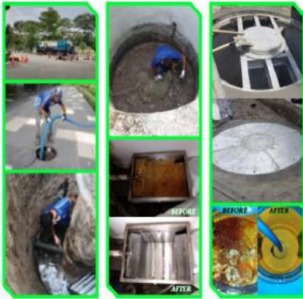
Using High Pressure Vacuum Of Grease Trap & Human Waste. Repair & News Installation Of Grease Trap & Covers
