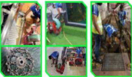
EM Rodding for clearing Choke and Floor Traps pipe maintenance
