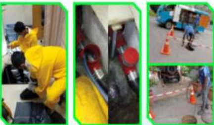
Using High Pressure water jetting for flushing of Manhole Over head pipes and grease traps
