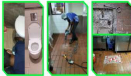
Dismanting of toilet & Urinal Bowls, Replacement of tiles
